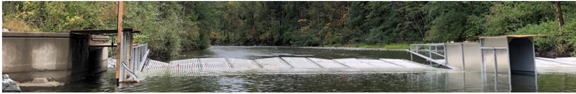
Figure 6: Two-passage counting fence configuration with wide passageways located mid-river and at the bulkhead, first piloted in 2019.
