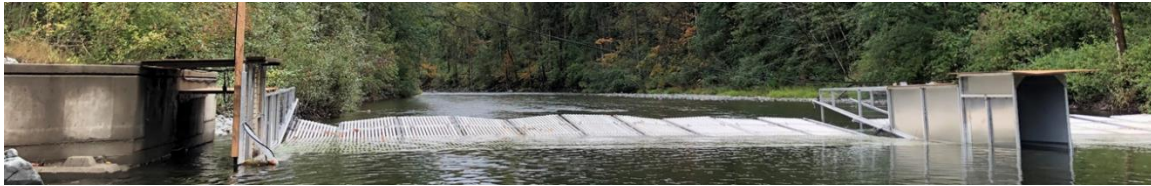
Figure 6: Two-passageway counting fence configuration with wide passageways located mid-river and at the bulkhead, first piloted in 2019.
