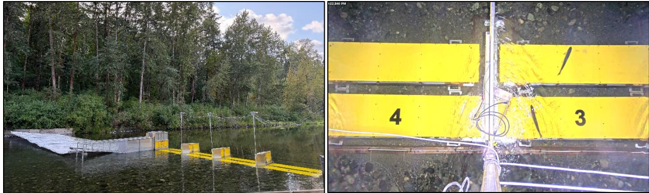
Figure 4: Traditional two-passage counting fence design used since 2019 (top) compared to the low-flow design with four open passageways and overhead camera views (bottom).
