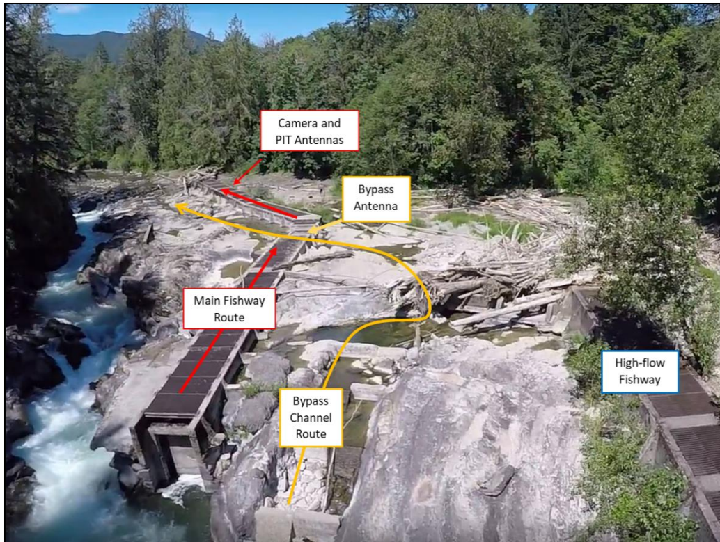
Figure 5: Skutz Fishways, bypass channel, migration routes, and monitoring equipment.
