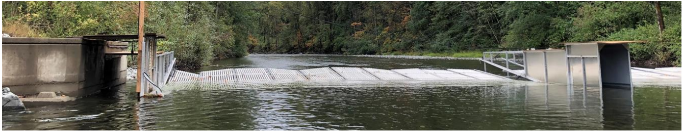
Figure 7: Two-passage counting fence configuration with wide passageways located mid-river and at the bulkhead, first piloted in 2019.
