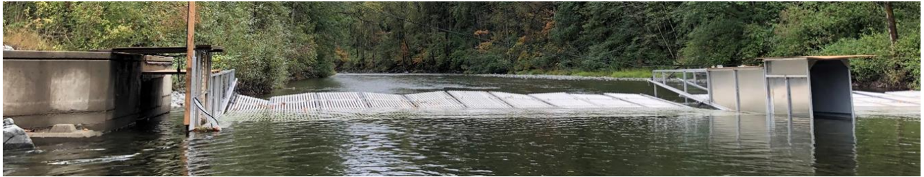
Figure 5: Two-passage counting fence configuration with wide passageways located mid-river and at the bulkhead, first piloted in 2019.
