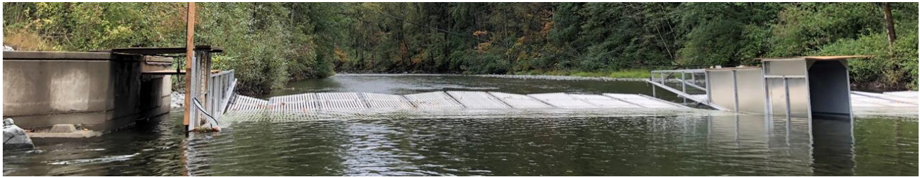
Figure 4: Two-passage counting fence configuration with wide passageways located mid-river and at the bulkhead, first piloted in 2019.
