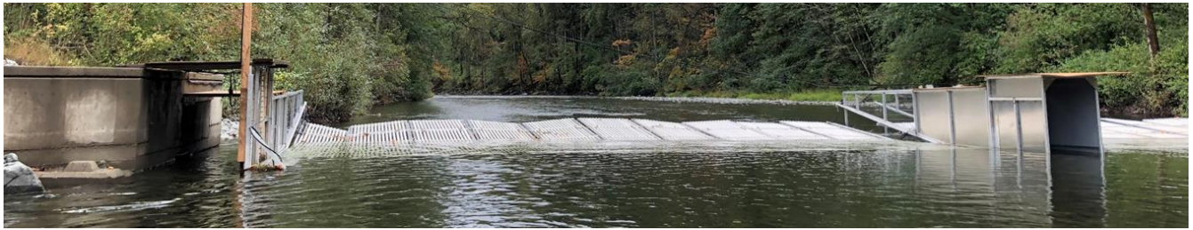
Figure 8: Two-passage counting fence configuration with wide passageways located mid-river and at the bulkhead, first piloted in 2019.
