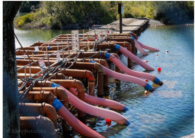
The Cowichan River needed electric pumps to keep water flowing for three weeks in 2019. Photo by Barry Hetschko.
