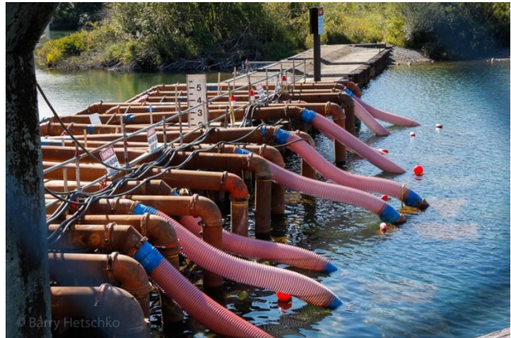
The Cowichan River needed electric pumps to keep water flowing for three weeks in 2019. Photo by Barry Hetschko.
