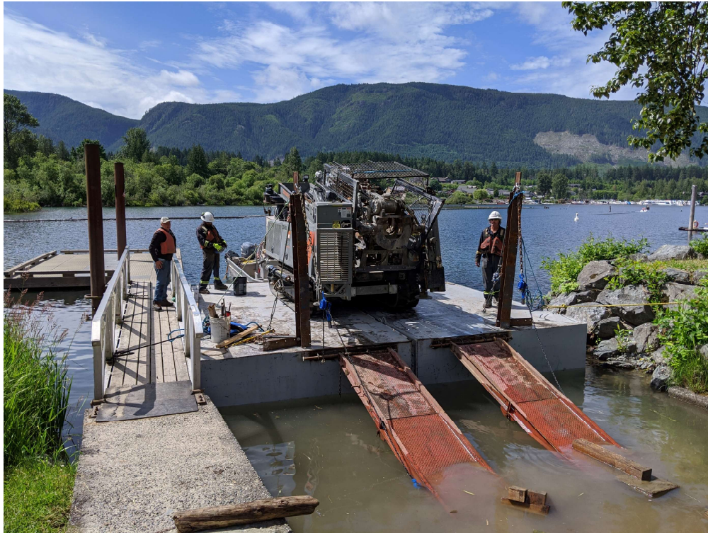
Drill Rig on Barge
