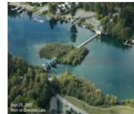
The weir is a cement structure, spanning Cowichan Lake at the head of the river. It includes a boat lock (at far right, above) and several 'spill gates' (left of the island).
