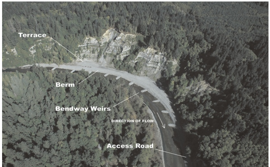
Figure 3. Stoltz Bluff berm, terrace, and bendway weirs in summer of 2007, one year after construction.
