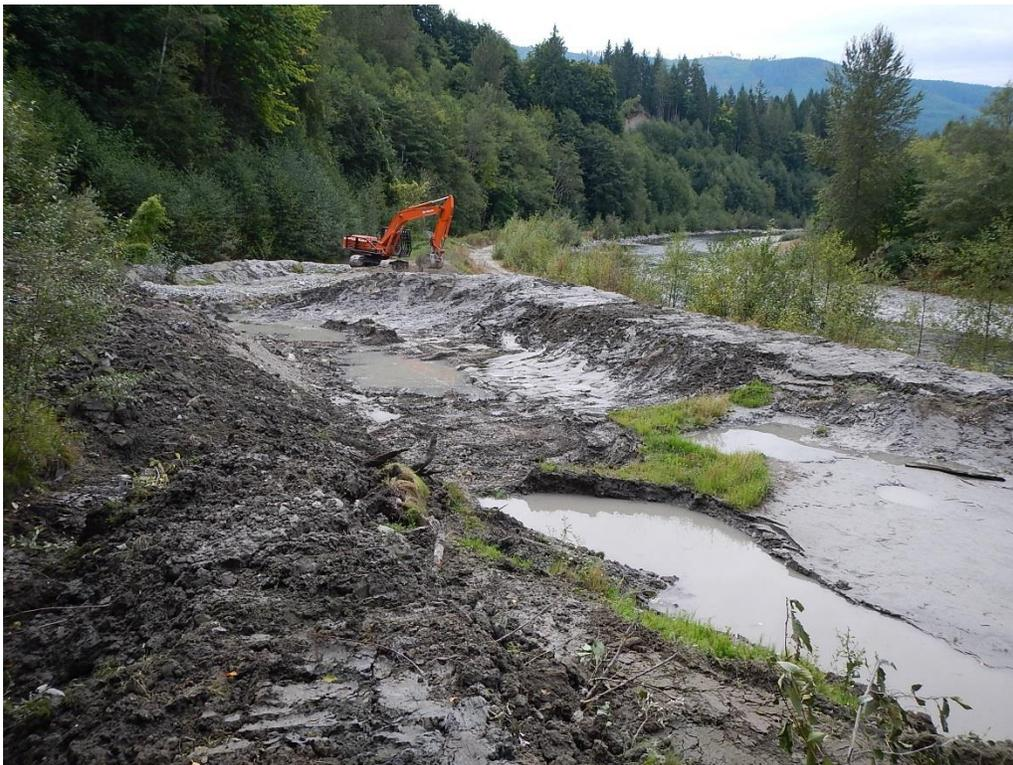
Figure 4. View looking downstream of primary sediment basin and uppermost check dam, near the end of maintenance excavation on September 17, 2014.
