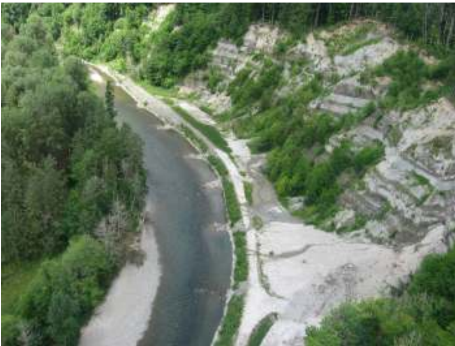
Stoltz Bluff Remediation project, June 24, 2010.
