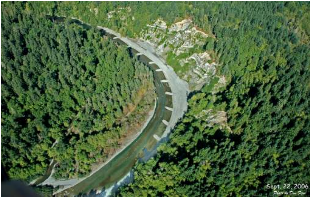
Stoltz Bluff Remediation project – Phase 1 complete, September 2006.
