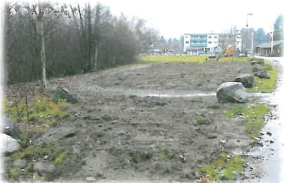
Grass removal and soil preparation for upland riparian planting
