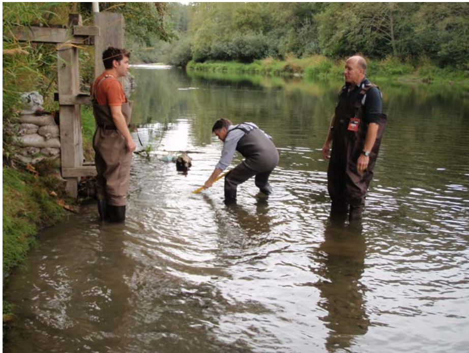
Figure 3 Installation of pressure transducer in the Cowichan River
