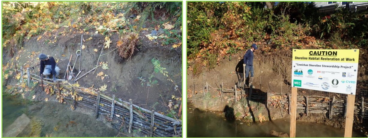
Figure 6. Construction of a live-stake wattle fence at a CSSP 2017 site along Cowichan River.
