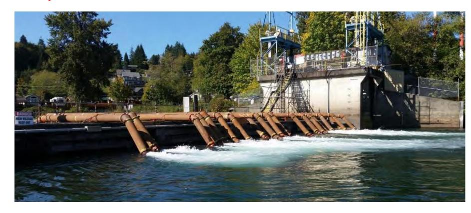
Pumps within screened box – small fish in area not evidently impacted by running pumps and at no risk
